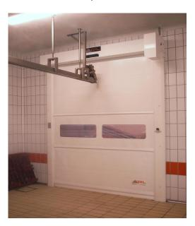
Retractable air block box between controlled atmosphere environments
